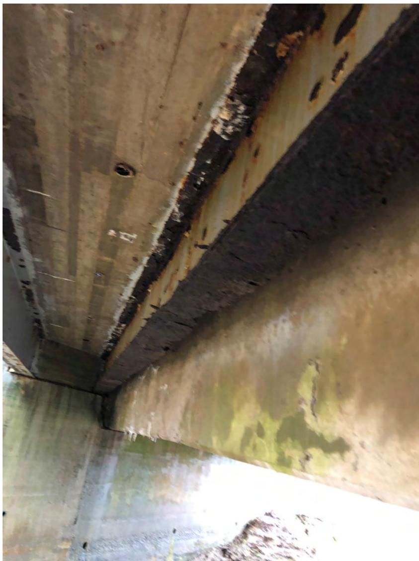
Extensive Corrosion of inner I-Beam at Inlet
