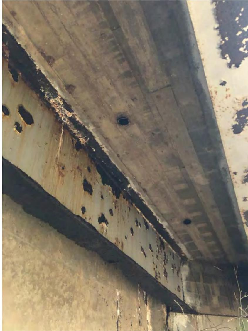
Extensive Corrosion on I-Beams at Inlet
