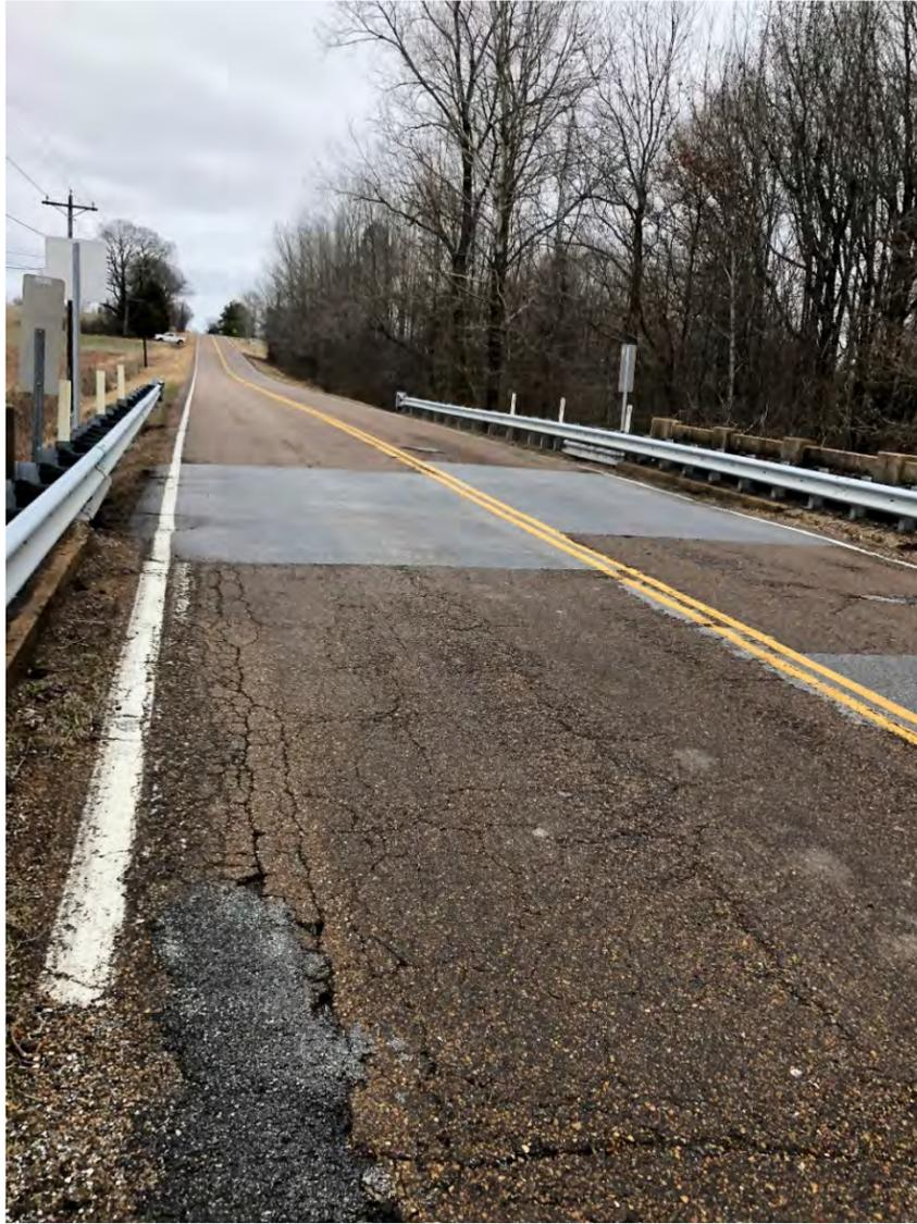
Pavement Cracking and Spalling along Surface from West Abutment
