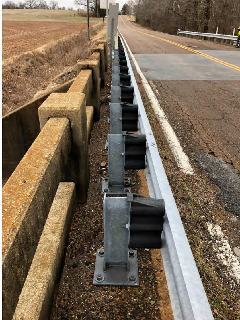
Poor conditions of Railing and Shoulder (Vegetation and Decay)
