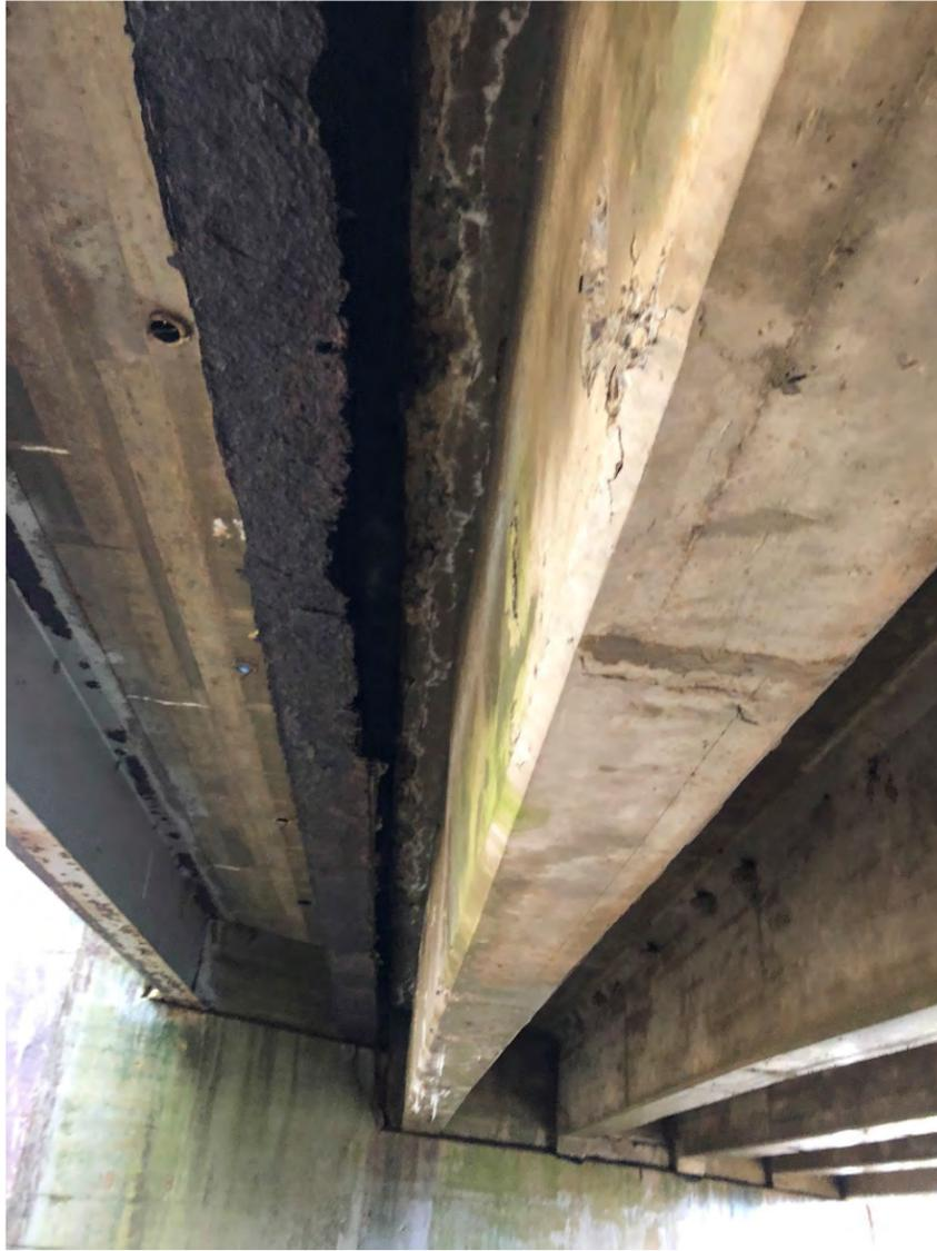
Extensive Corrosion of inner I-Beam at Inlet
