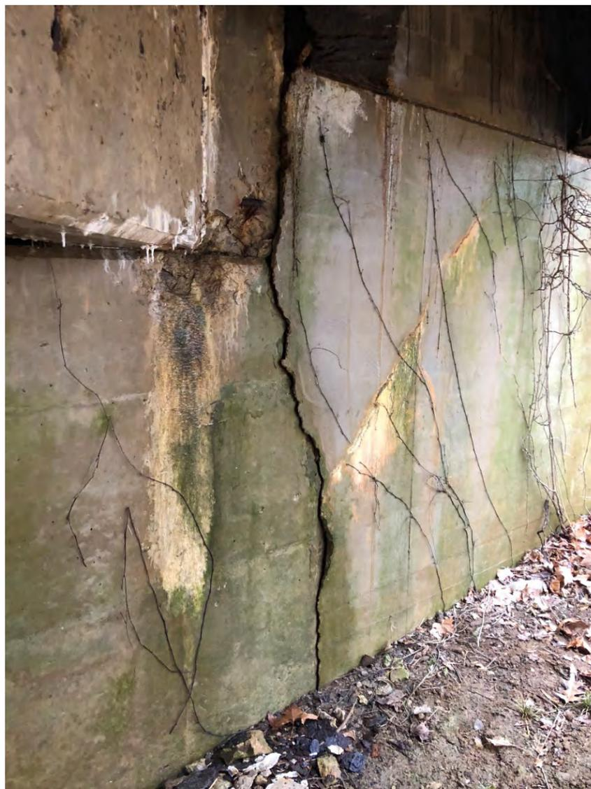
West Abutment Decay and Cracking
