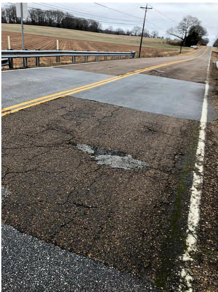
Spalling and Cracking along Surface
